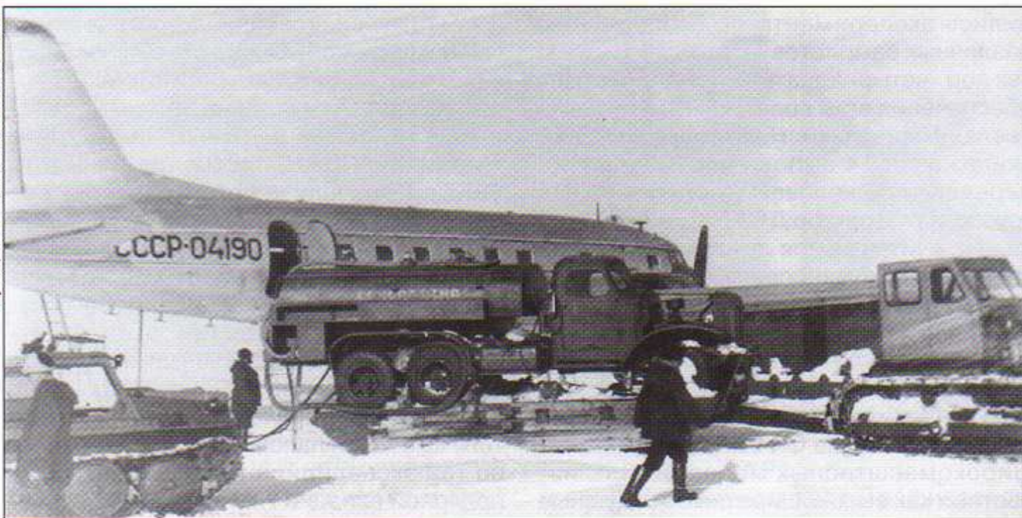
Заправка топливом от перетаскиваемого на специальных санях автозаправщика The aircraft is being refueled from a refueller, which is carried on special sledge
